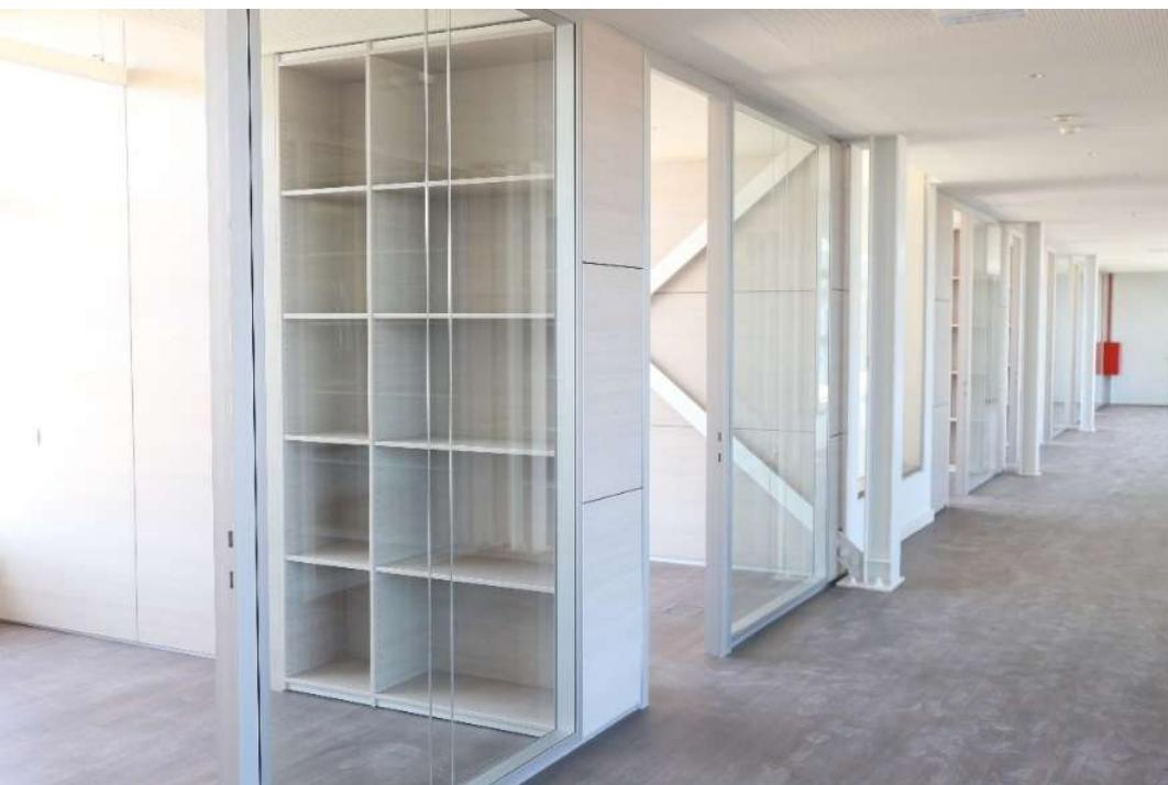
Double glass partition walls integrated with opaque walls.
